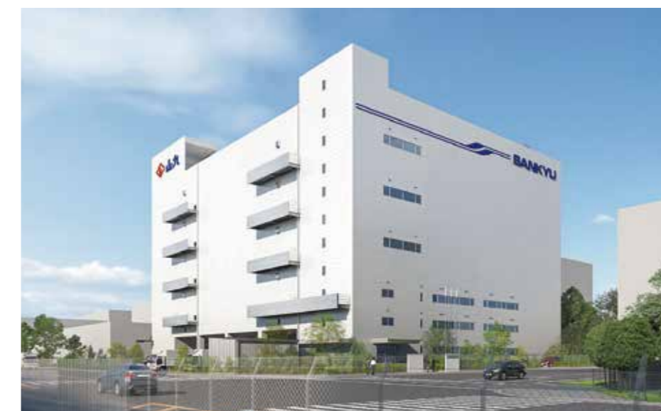
In April 2023, the Odaiba Logistics Center was opened in the Odaiba area of Koto-ku, Tokyo.
